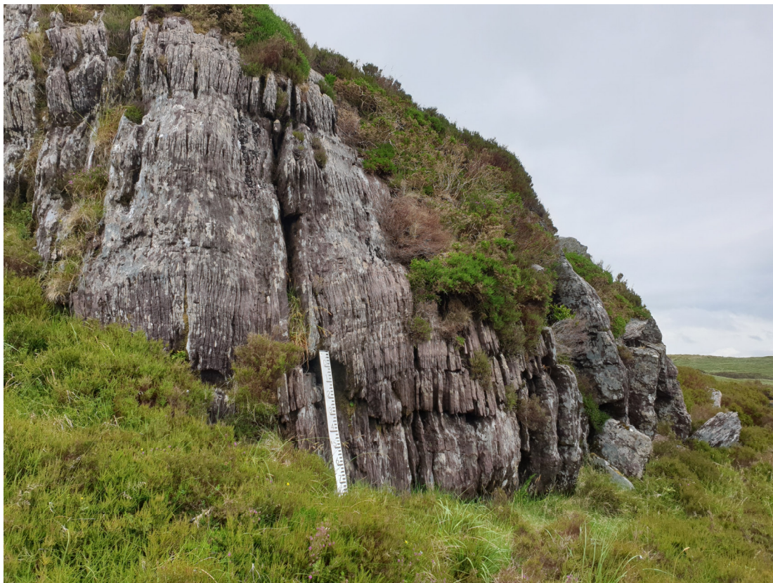
Exposed and weathered bedrock outcrop observed during site survey 18/06/2020.
